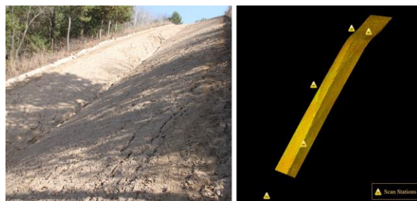
Figure 3 Five monitoring stations
